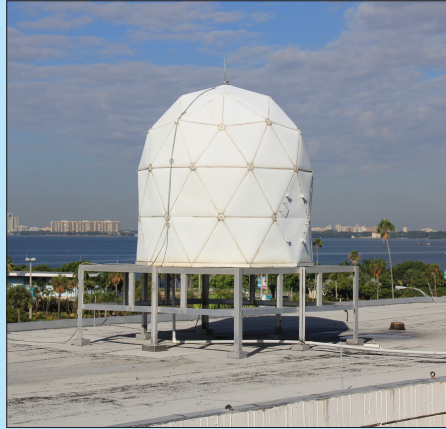
Perched on the roof at AOML, a protective radome covers a 1.7 m satellite receiving station.
