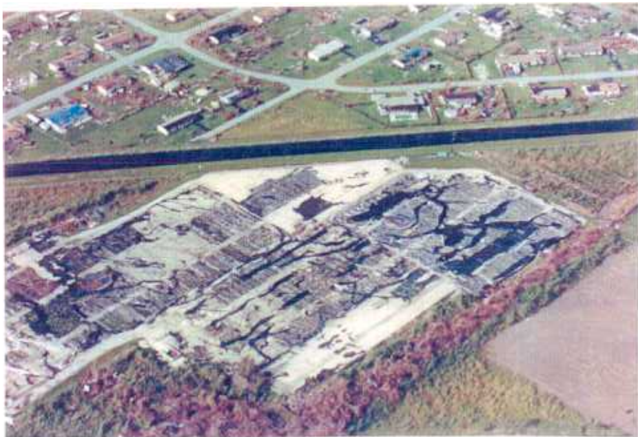
23. Damage to nursery and adjacent housing.
