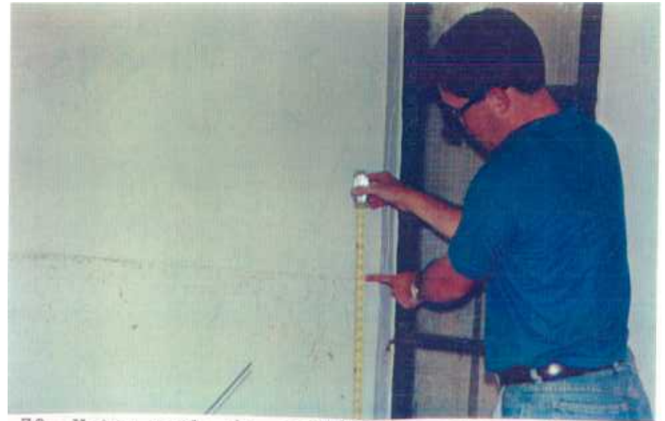
70. Water mark in residence along Old Cutler Road south of Coral Gables.
