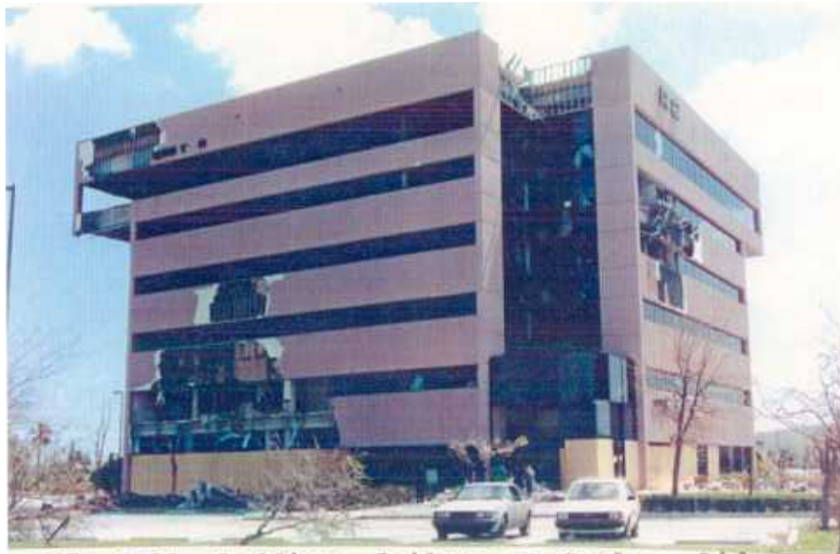
67. Wall cladding failure at Cutler Ridge office building.
