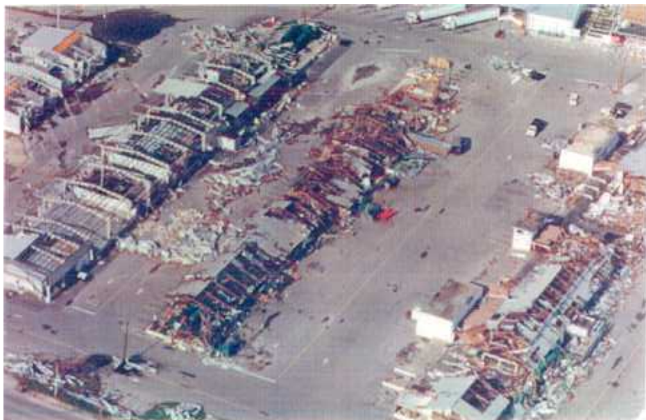
7. Loss of cladding and several collapsed bays in metal buildings along Highway 1.
