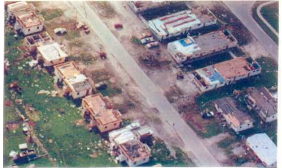
18. Flat roof damage (to F2) on multi-family dwellings in Florida City. View looking southeast.
