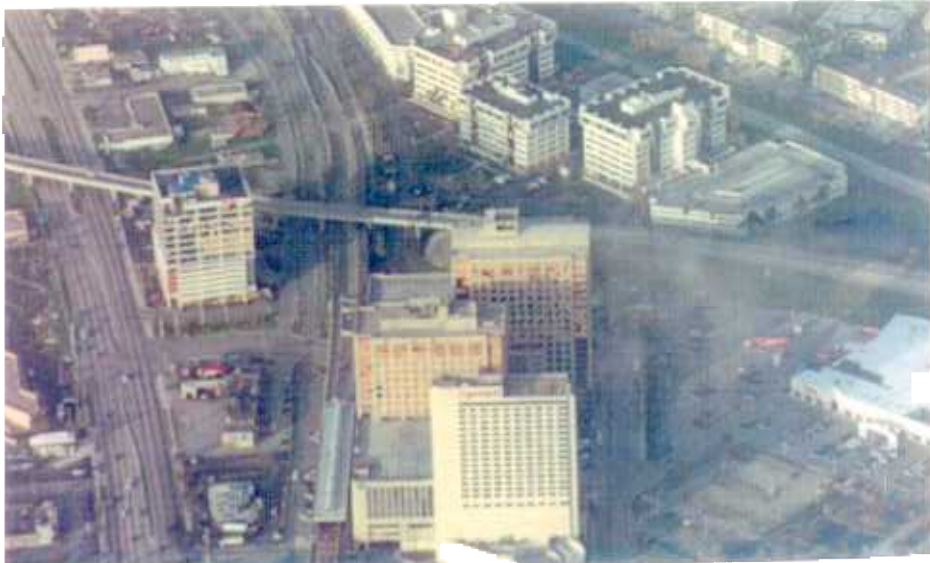
1. Broken window glass (boarded windows) downwind of Marriott Hotel in Coral Gables. View looking south-west along Highway 1.
