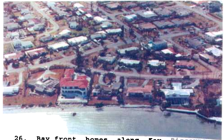
26. Bay front homes along Key Biscayne remained intact. Only minor roof and surge damage was noted.
