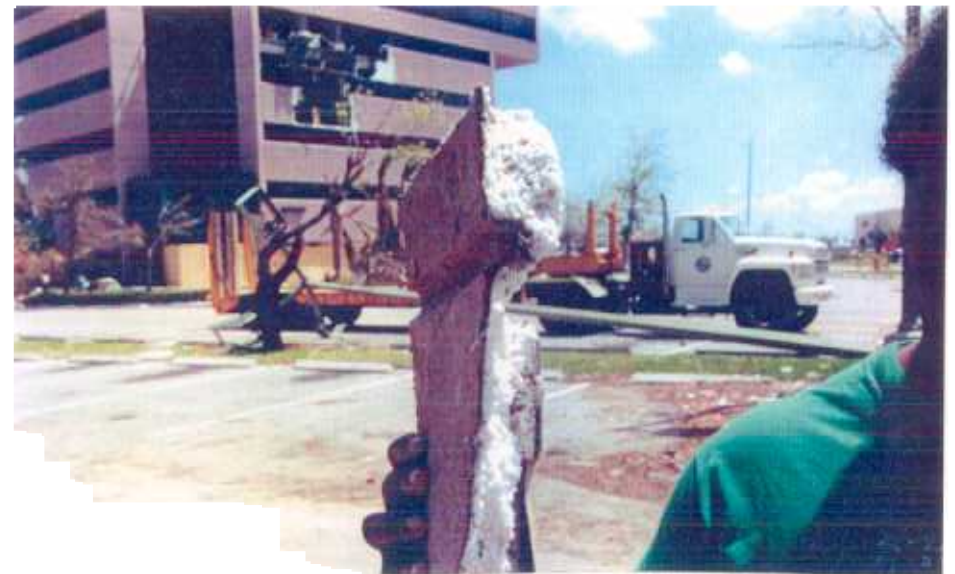
68. Cladding was composed of stucco type finish over a fabric mesh that was bonded to styrofoam insulation.
