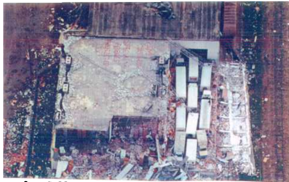
8. Collapsed north and west walls of concrete masonry building housing Budweiser Distributing .
