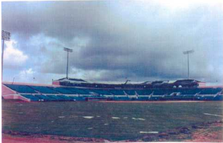
57. Cleveland Indians stadium in Homestead Florida. Light standards remained upright.
