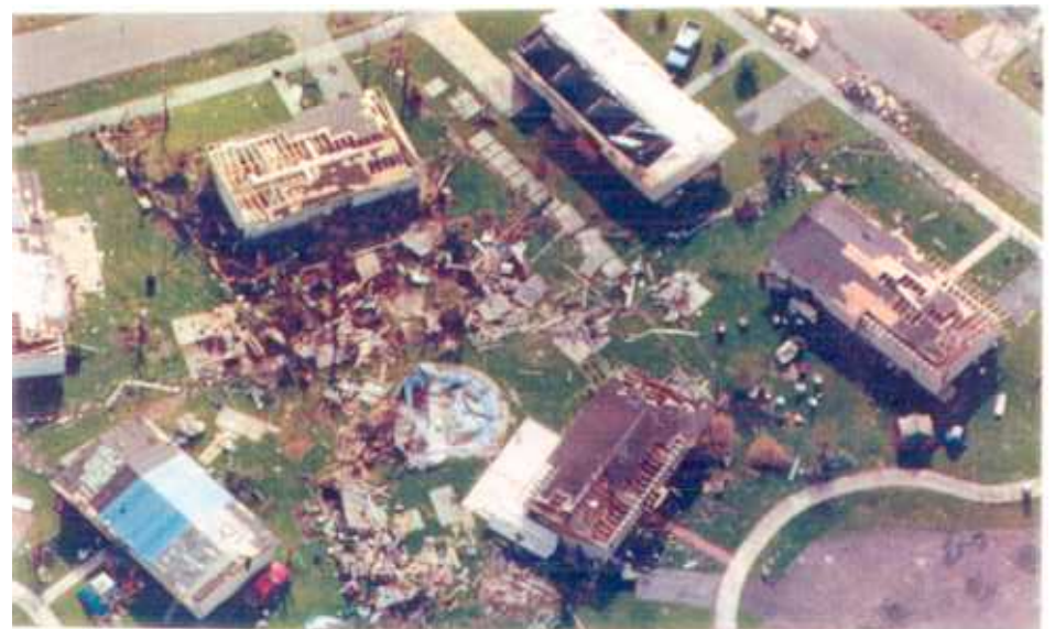
16. Removal of roof deck exposed wooden trusses on concrete masonry homes in Florida City.
