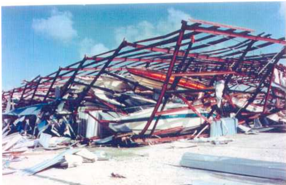
73. Two story steel boathouse collapsed crushing boats at Black Point Marina.
