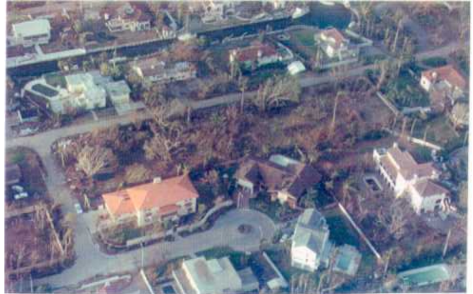
2. Minor roof damage to residences in Coral Gables.
