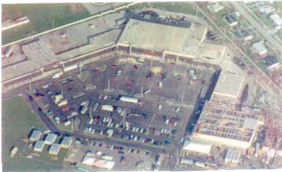
3. Partial loss of roof and metal decking in shopping center along Highway 1 near Perrine. View looking northwest.
