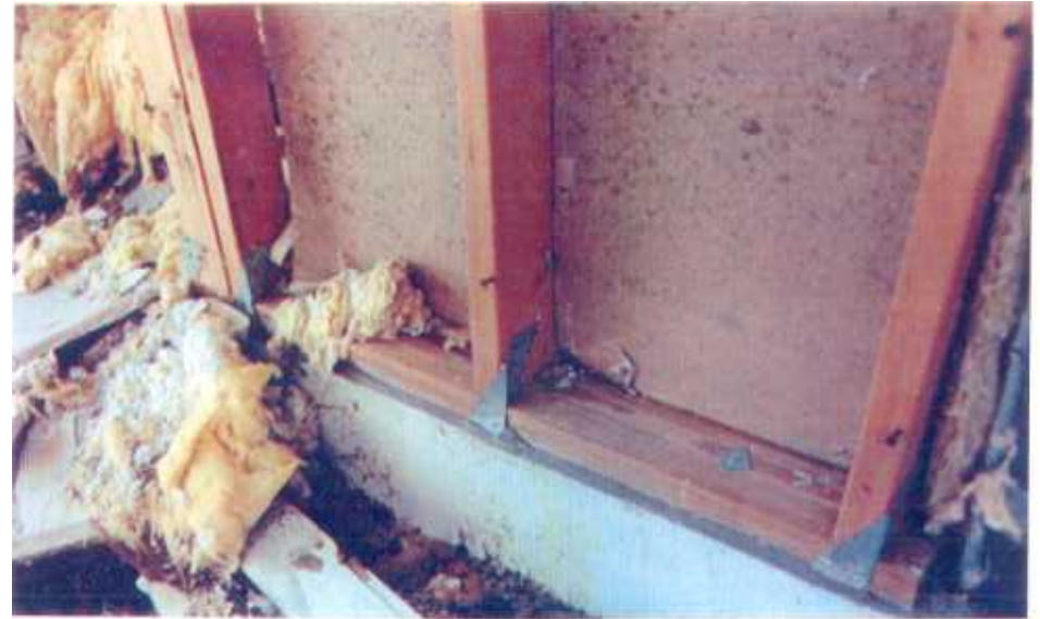
46. Metal clips secured wall studs to bottom plate. The bottom plates were nailed into the foundation.
