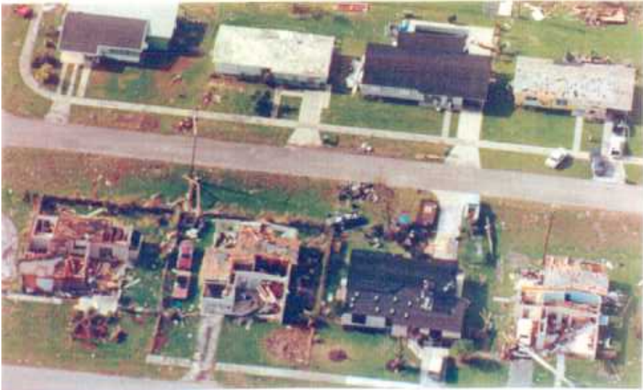
17. Residence damage (F0 to F2) which likely initiated in carport area. View looking south in Florida City.
