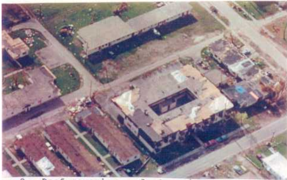
9. Roof covering lost in opposite directions on Florida City apartment building (looking southeast).
