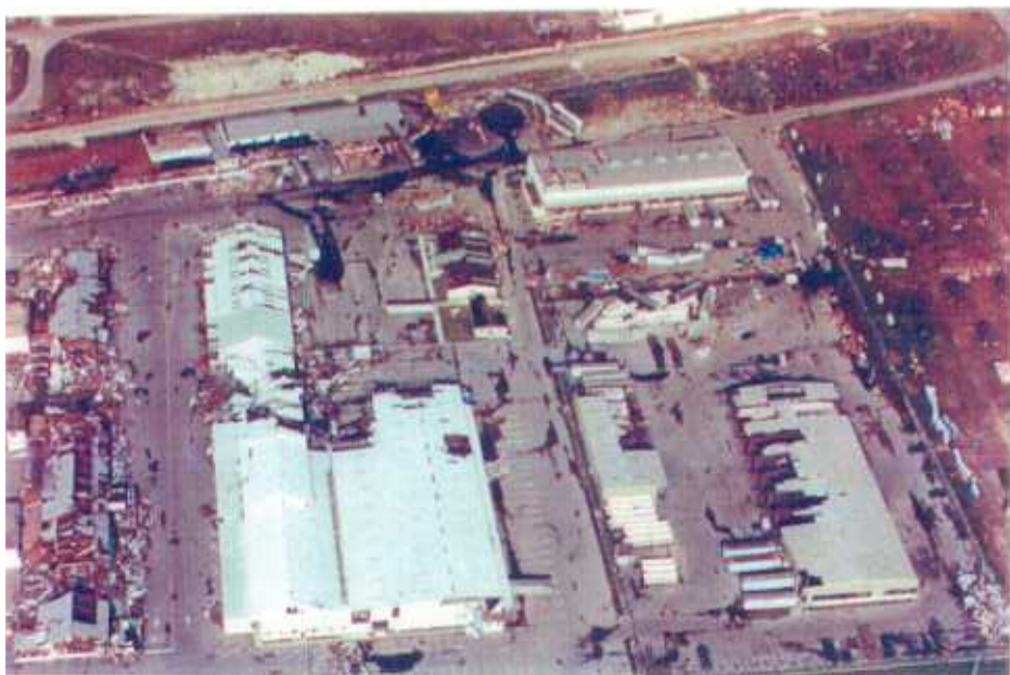
5. Metal building damage along Highway 1. View looking west.
