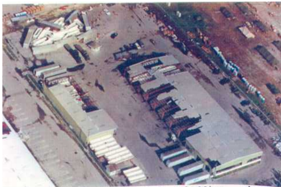
6. Loss of metal roof cladding above loading bay doors. View looking northwest.
