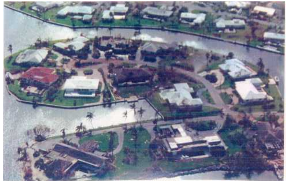
24. Minor roof damage to homes in Ocean Reef community on Key Largo.
