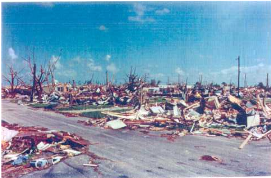
49. One of several destroyed mobile home parks in Homestead.
