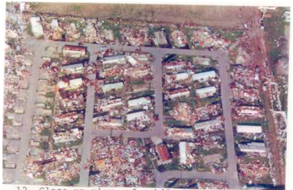
12. Close-up view of mobile home park in Homestead. View looking west.
