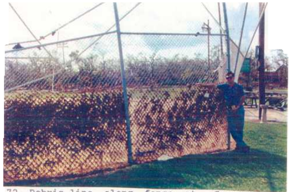
72. Debris line along fence at Coconut Grove Marina.
