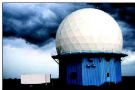
Norman, Oklahoma, Doppler radar installation.
