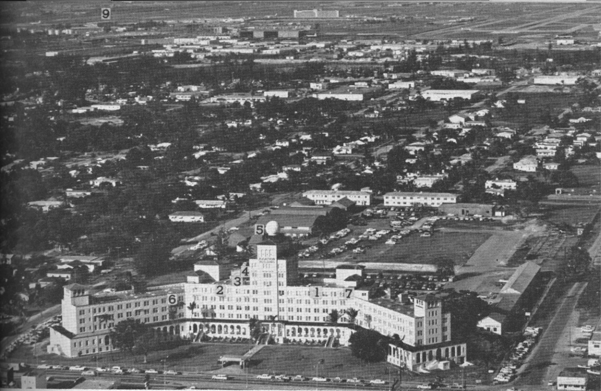
FIG. 1. Home of the National Hurricane Center, The Aviation Building, Miami, Florida—1. 5th Floor, North Wing, Hurricane Forecast Center—DMO. 2. 5th Floor, South Wing, NHRP Headquarters. 3. Offices of Research Flight Facility. 4. 7th Floor, Joint Facilities—Library—Conference Room—Drafting—Film Reading—Radar Maintenance—Research. 5. WSR-57 Radome. 6. Navy Fleet Weather Facility. 7. Project Mercury Support Group. 8. American Airmotive Facilities at Miami International Airport where research planes are housed and maintained. 9. Weather Bureau Airport Station, Miami. All of these establishments contribute in greater or lesser degree to the National Hurricane Center.
