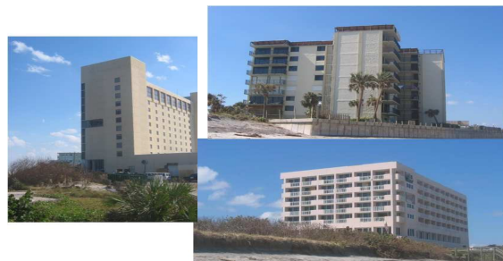
Figure 13. Examples of mid- and high-rise buildings.
