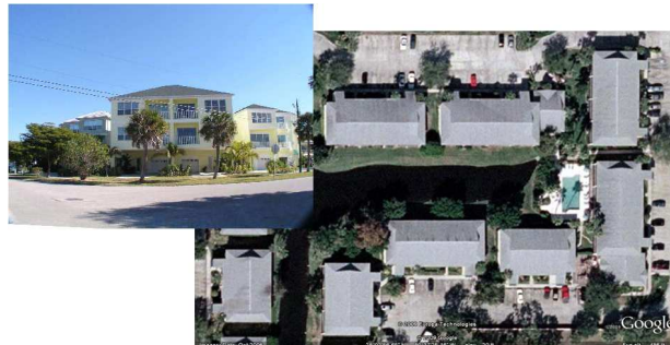
Figure 12. Typical low-rise buildings.
