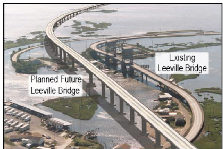
Figure 25.5. This “mock-up” shows the existing Highway LA-1 and Levee Bridge in coastal Louisiana (on the right) with a planned new, elevated bridge that would retain functionality under future, higher sea level conditions (center left). (Current sea level and sinking bridge are shown here.) A 7-mile portion of the planned bridge has been completed and opened to traffic in December 2011. (Figure source: Greater Lafourche Port Commission, reprinted with permission).
