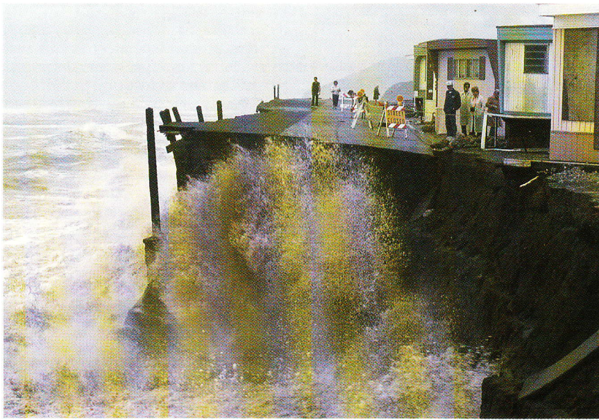
Figure 12 Damage due to coastal erosion by high surf at Pacifica, near San Francisco, California in 1983. (Photo by James Sugar/Black Star.)
